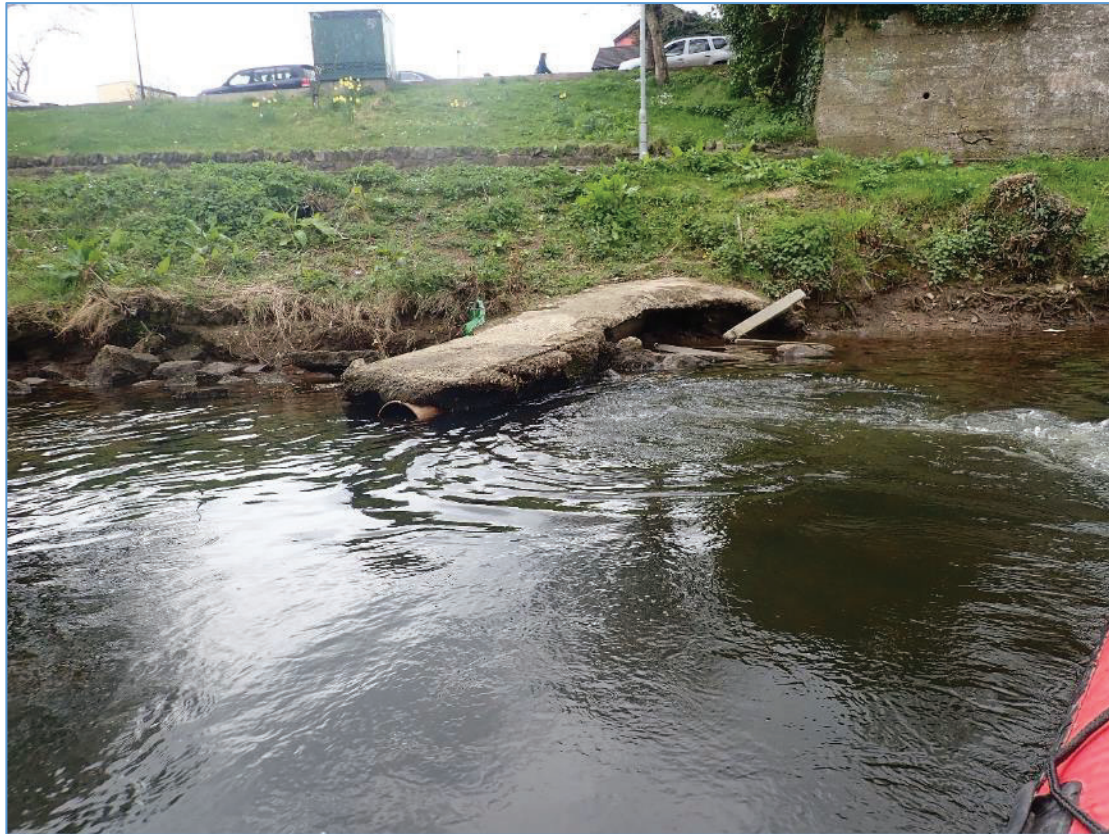
Plate 17: Outfall entering the river from the south bank above Arklow Bridge.
