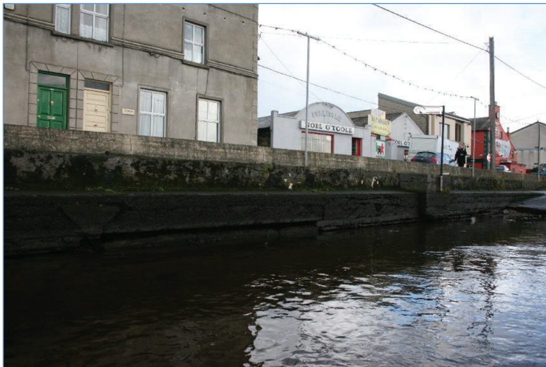
Plate 31: View along South Quay showing the stone wall and later concrete additions.
