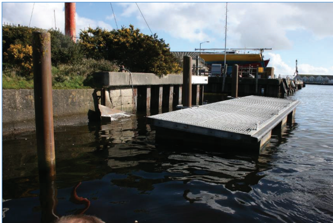
Plate 27: At the marina, the concrete caissons are replaced by sheet-piling capped with a concrete deck.
