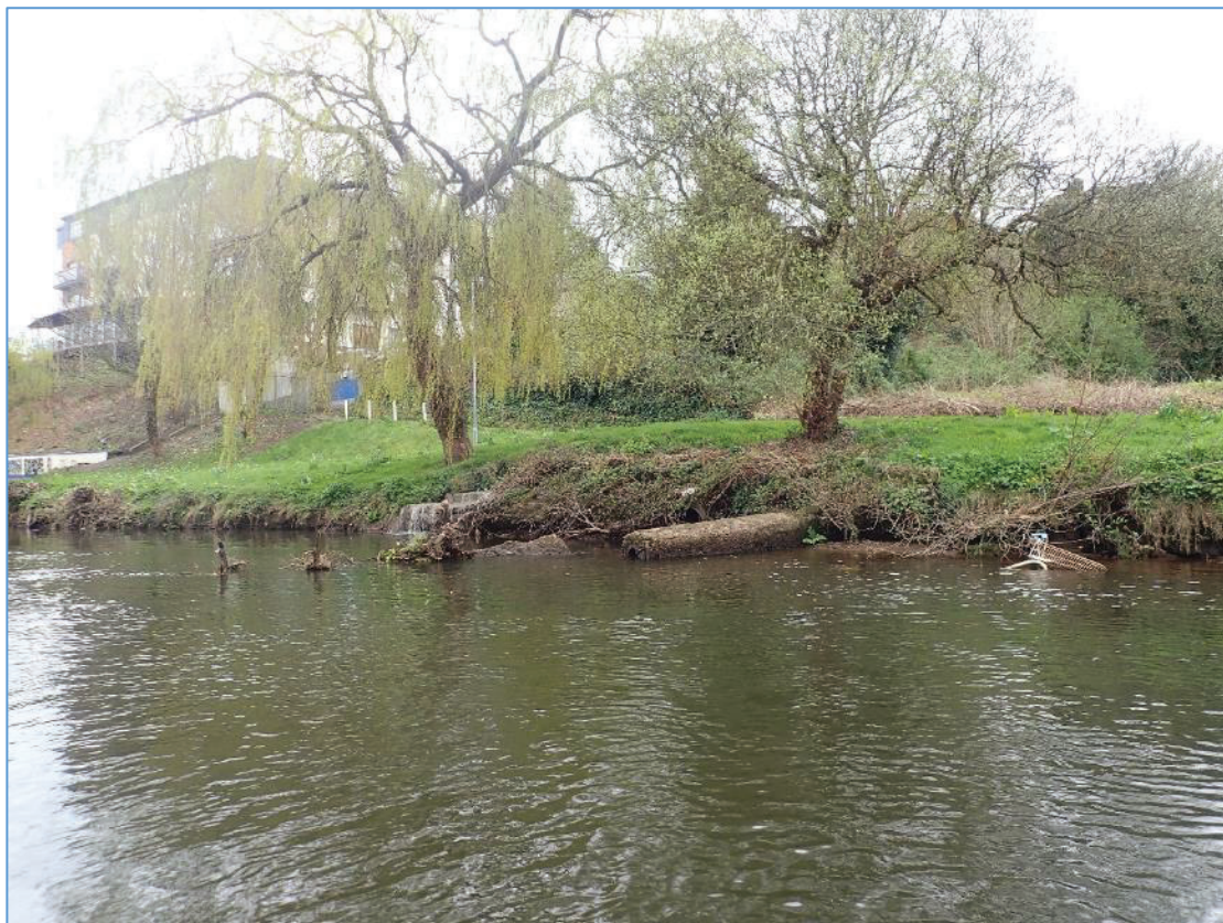
Plate 18: Outfall entering the river from the south bank above Arklow Bridge.
