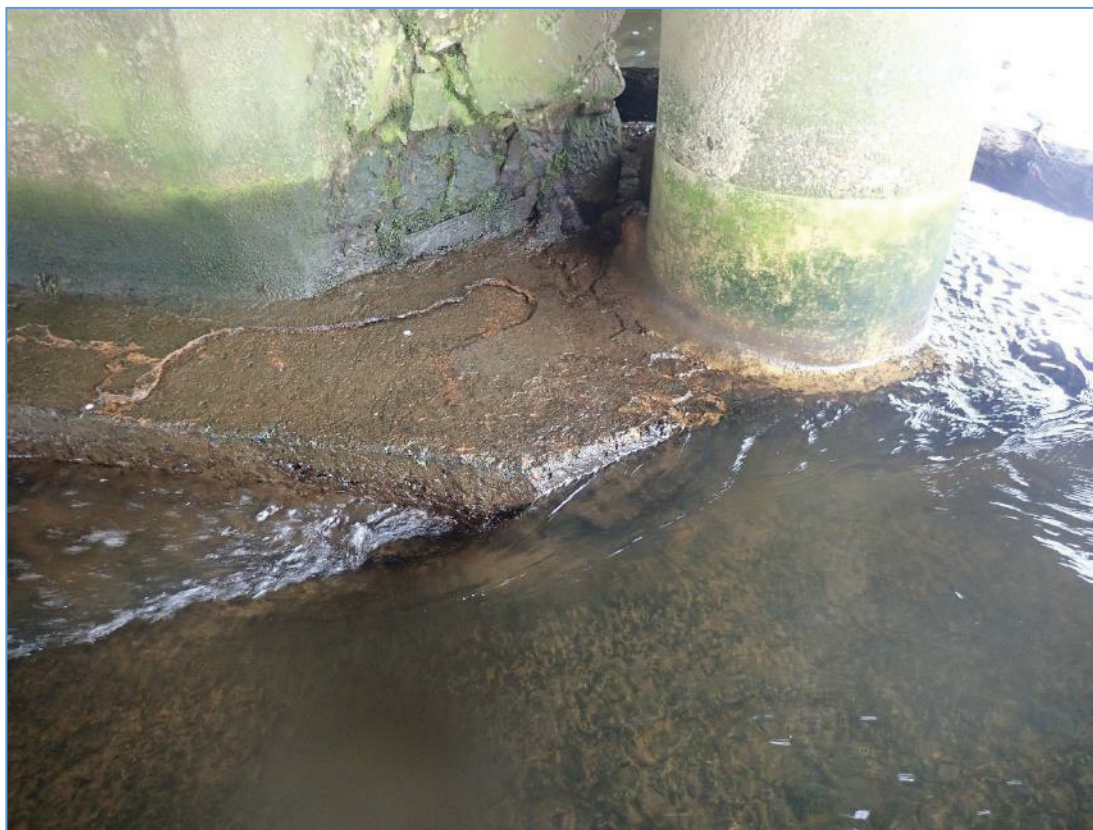
Plate 62: Detailed view of the junction of the 1960s work with the stone bridge.
