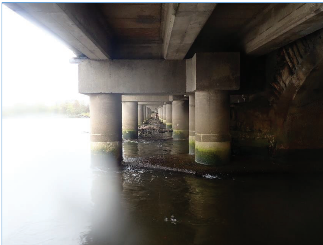
Plate 60: View looking North across the base of Arklow Bridge, showing the 1960s addition to widen the structure.
