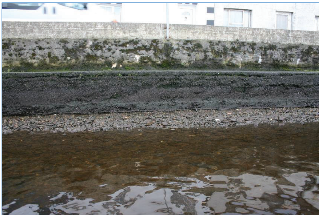
Plate 32: View of South Quay showing the stone wall and later concrete additions.
