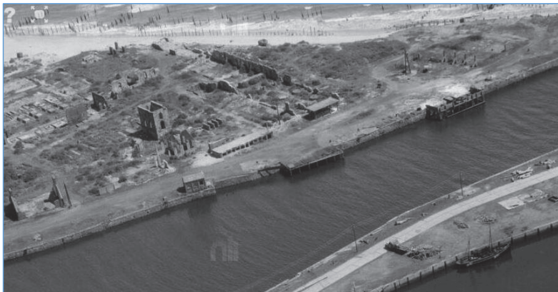
Plate 7: Arklow Harbour, the lower North Quay area showing the stone quayside in 1956. By Alexander Morgan. It is now replaced by sheet-piling. Source: National Library of Ireland.
