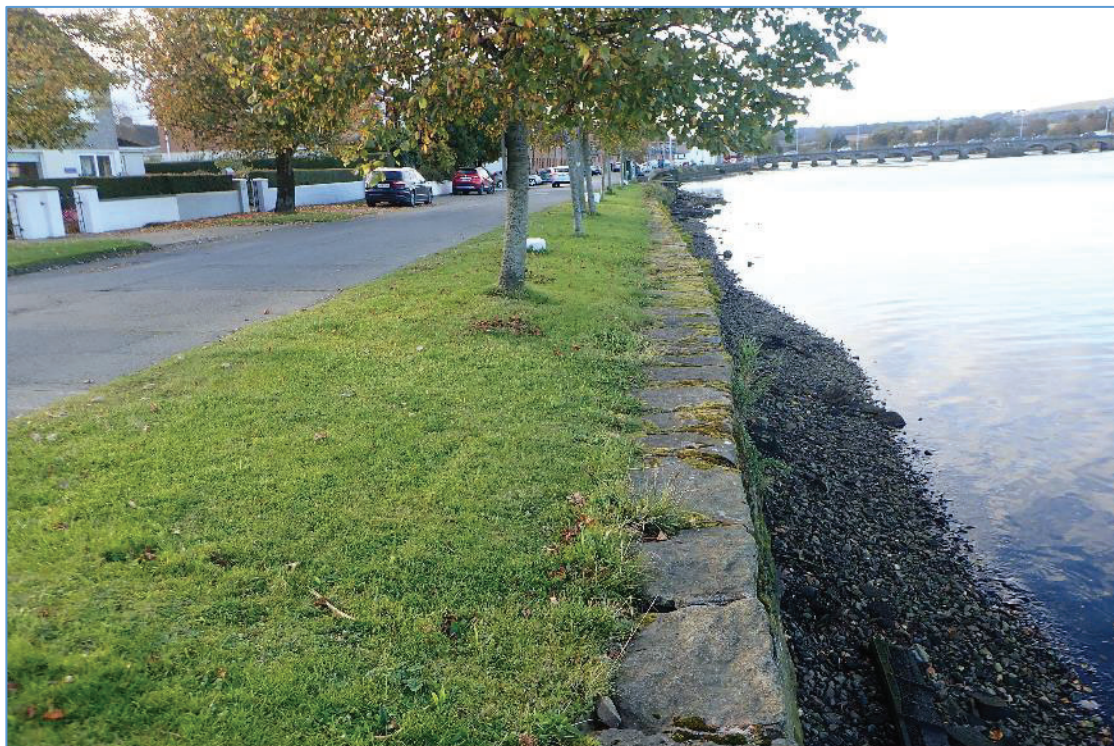
Plate 35: View on South Quay looking upstream showing the nature of the stone capstones that are part of the original stone structure.
