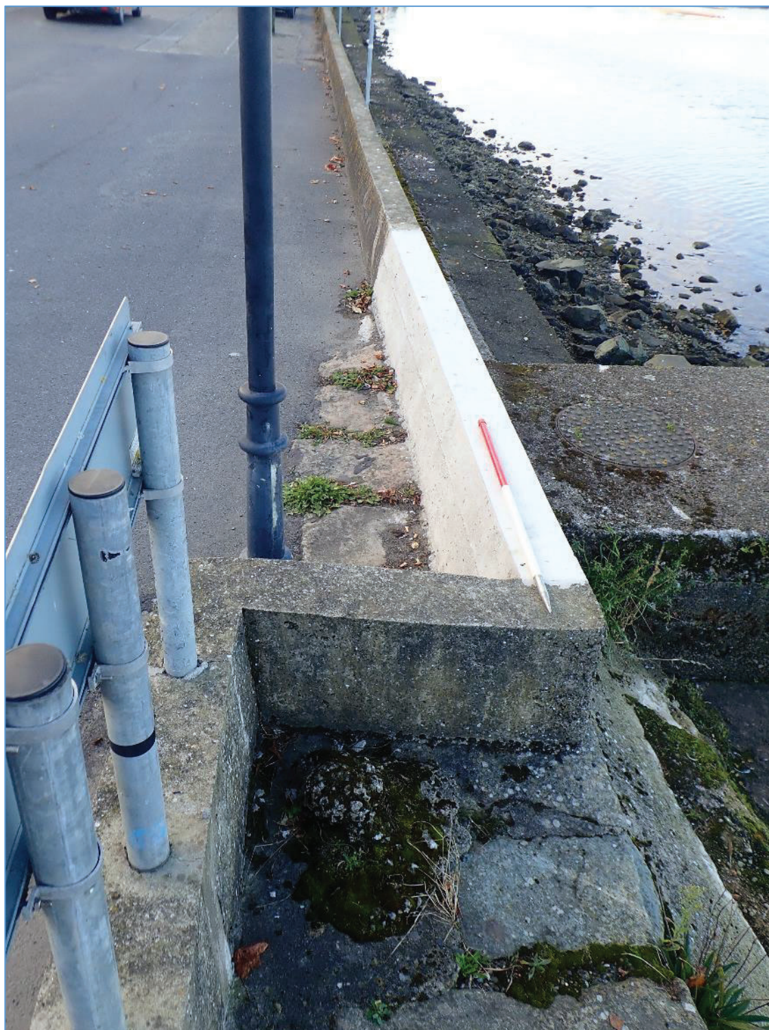
Plate 33: View on South Quay looking upstream from where the stone quay becomes buried under modern concrete.
