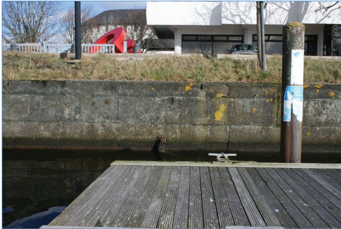
Plate 25: A concrete caisson solution marks the North Quay between the sailing club and the marina.
