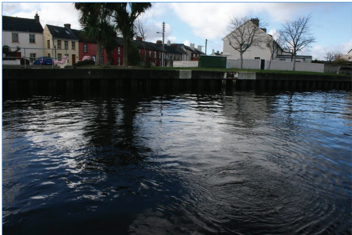
Plate 41: View of sheet-piling that defines the lower reaches of South Quay.
