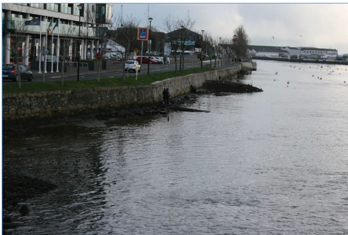
Plate 20: View downstream from Arklow Bridge at the stone retaining wall of North Quay.
