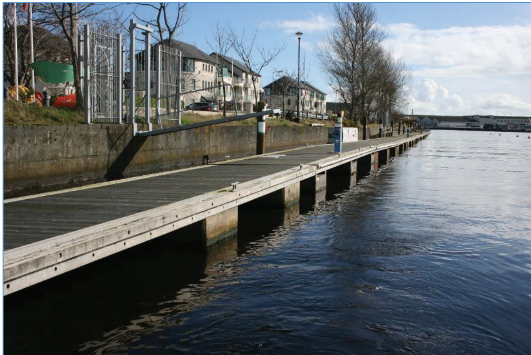
Plate 26: View along North Quay should galvanized gangways to access the floating pontoon.
