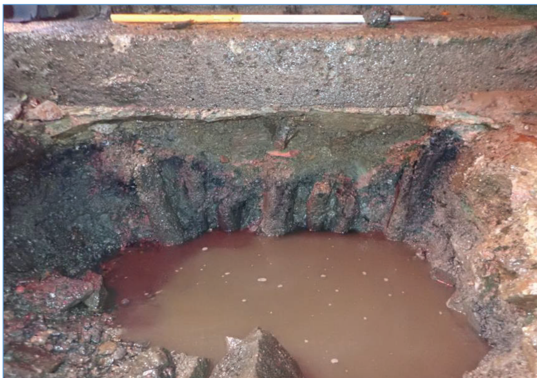
Plate 64: TP-04 at Pier 4. Excavation reveals a line of starling piles under the stone apron.
