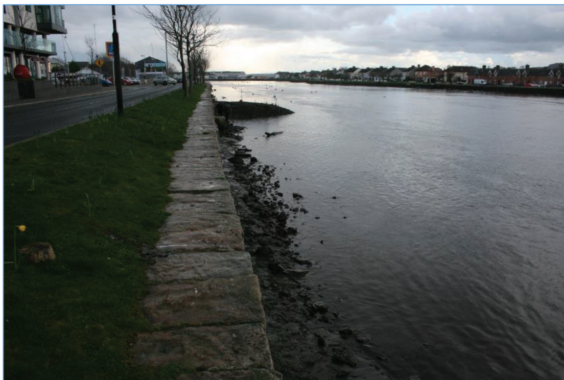
Plate 22: View looking downstream on North Quay, showing the granite capstones of the quay.
