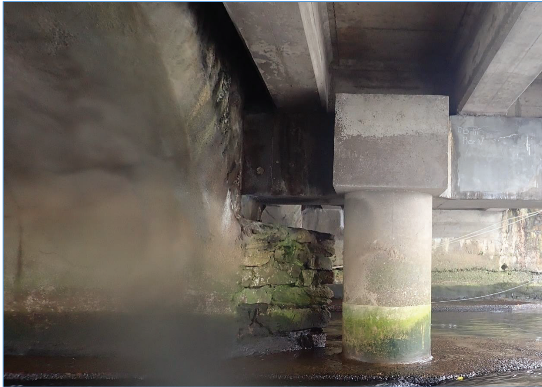
Plate 61: View looking South at the junction of the 1960s work with the upstream façade of the stone bridge.
