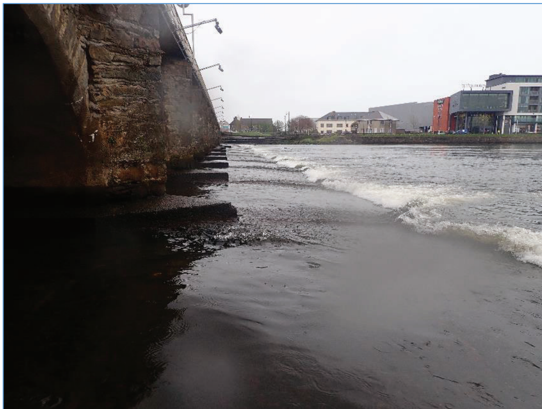
Plate 59: Stone scour apron added to the downstream side of Arklow Bridge, forming a glaciais feature.
