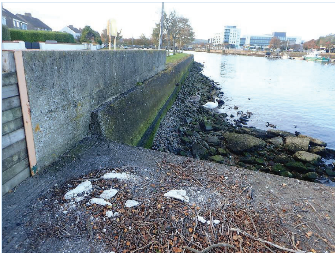
Plate 38: View from boatyard slipway looking upstream, showing the convergence of South Quay and its later concrete rendering.
