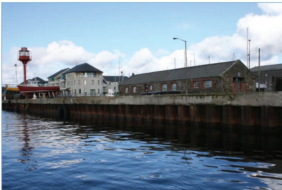
Plate 28: Sheet-piling now defines the remainder of the North Quay downstream of the marina.
