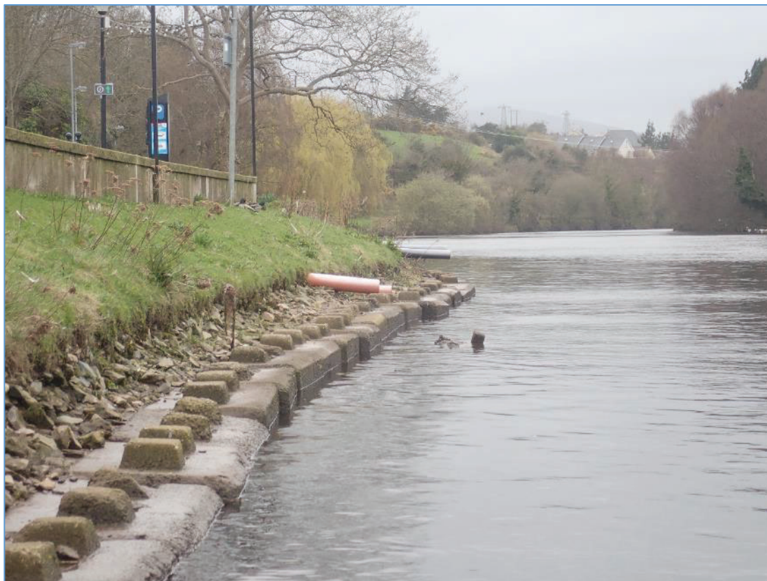
Plate 19: View looking upstream along the retaining measures at the Riverwalk.
