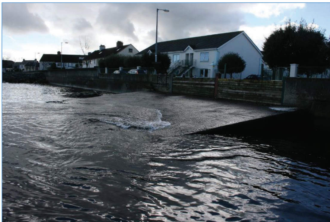
Plate 39: View looking southwest and downstream at the concrete-covered slipway that formerly served as the slipway for a boat-building yard that is recorded on the OS 1911 map.
