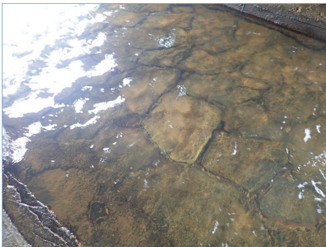
Plate 58: View of stone scour apron set between the bridge piers, Arch 19.
