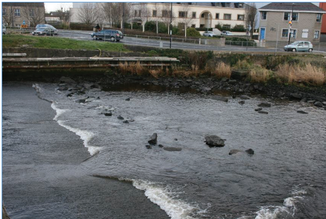
Plate 23: View looking across to North Quay, showing the service pipes to the former NET/IFI factory carried on the wall.
